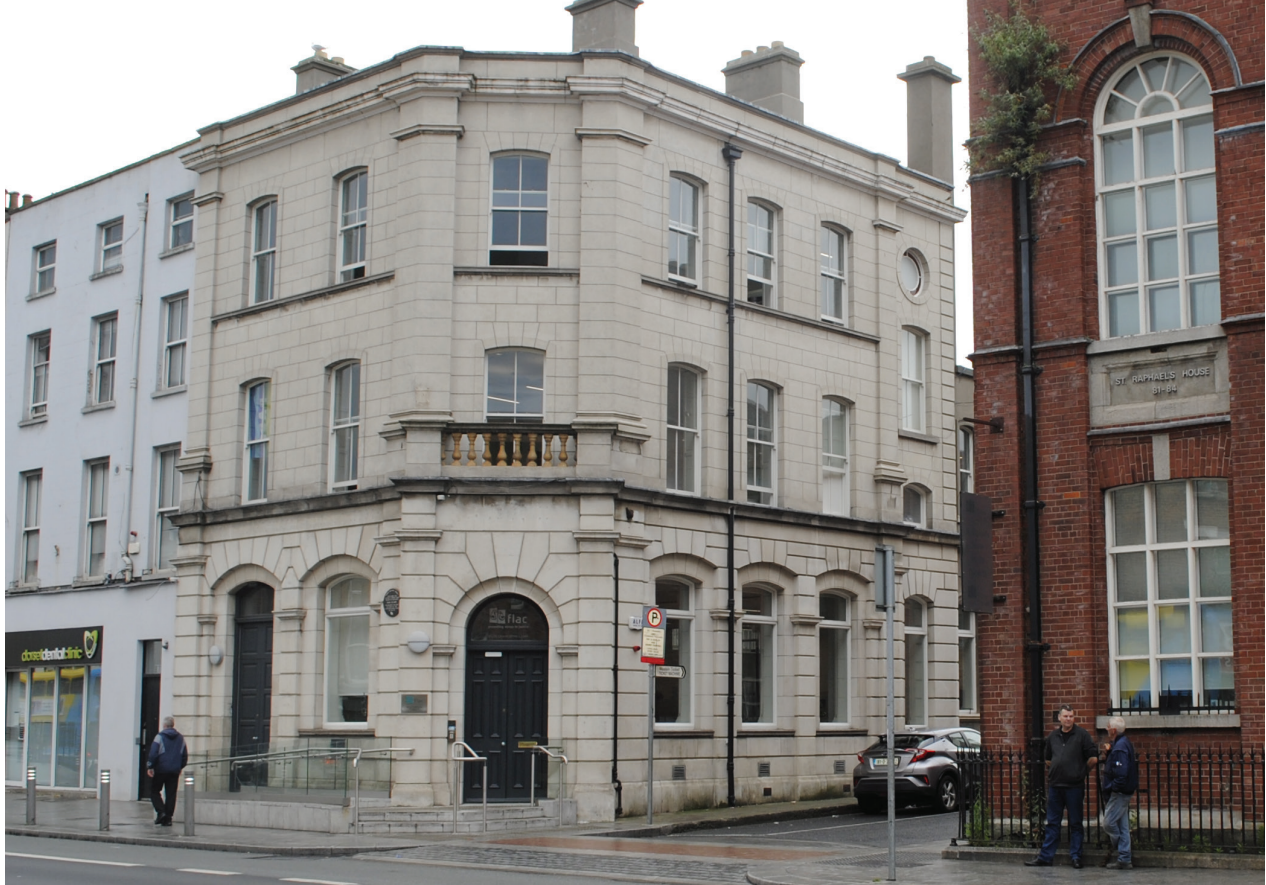
FLAC's Offices at 85/86 Dorset Street Upper.
